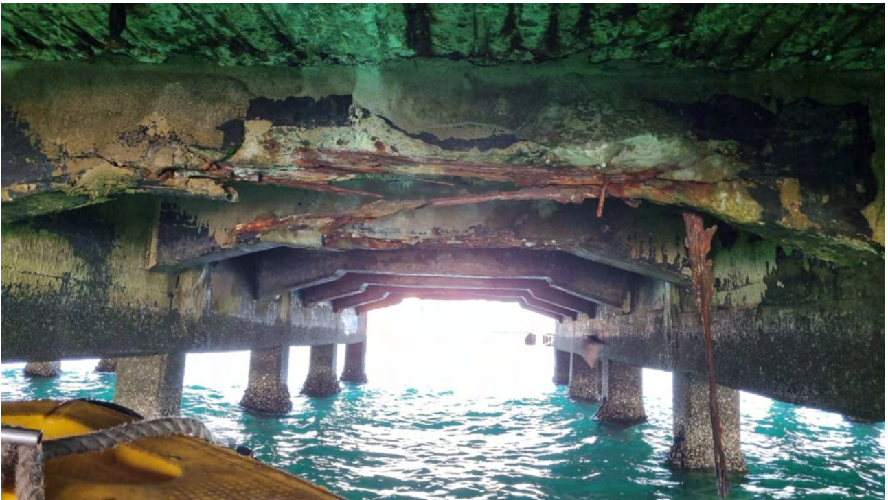
Figure 7: Public Wharf Cross Beams
