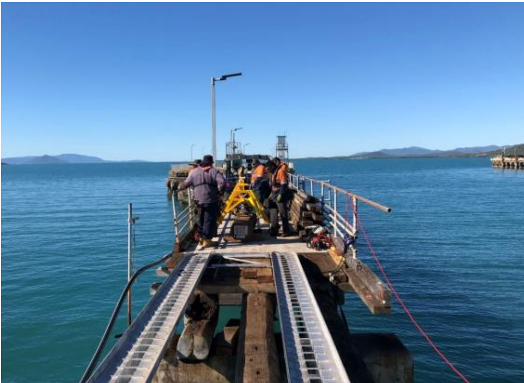
Figure 15: Jinker trailer assembly and access ramps (outer stem)
