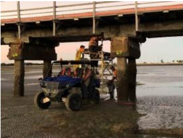
Figure 12: Example headstock access (note platform would need to be lowered to access base of headstock)
