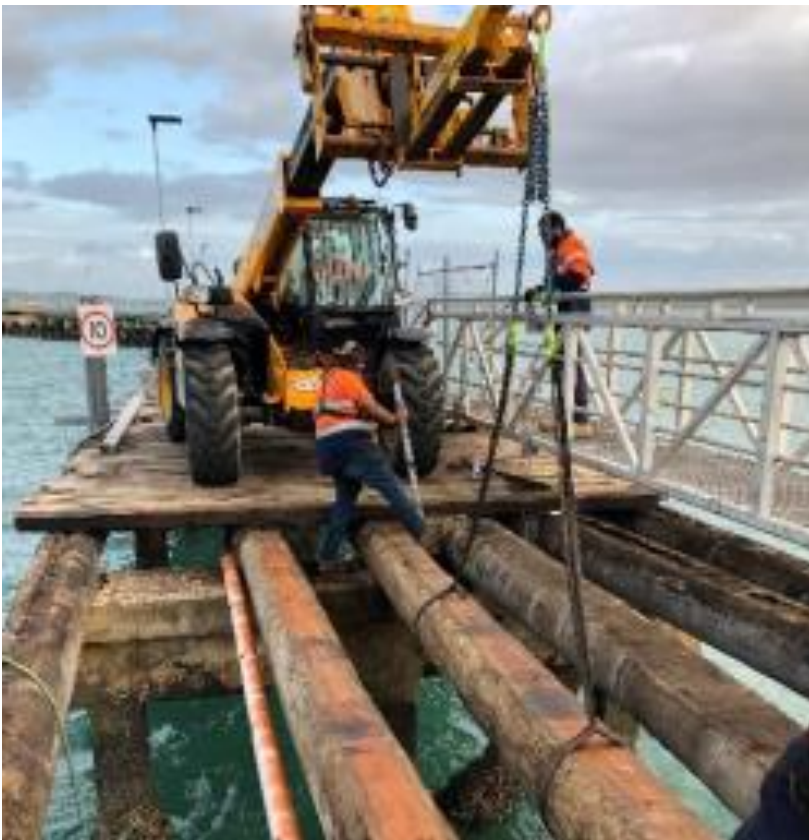
Figure 14: Girder replacement with a Telehandler (middle stem)
