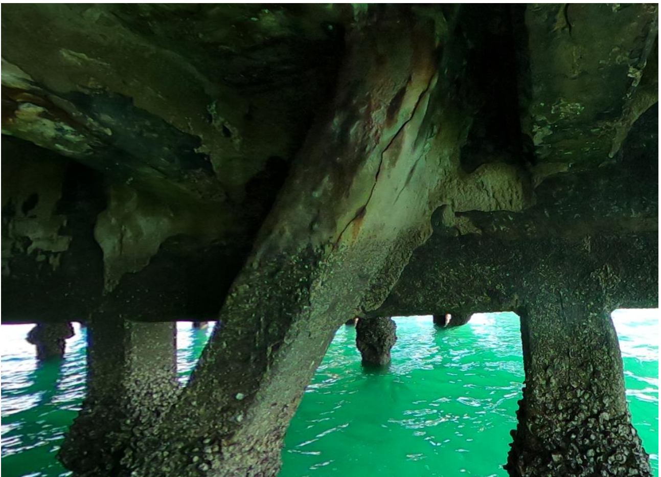
Figure 6: Public Wharf Piles (top)
