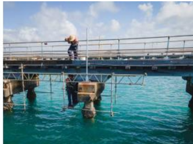
Figure 12: Example headstock access (note platform would need to be lowered to access base of headstock)
