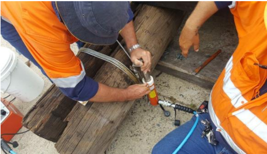
Figure 16: Type 2 Corbel Repair "Wire Wrap" Testing during Bowen Wharf Repair Project
