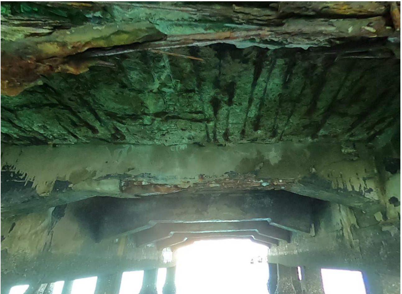
Figure 8: Public Wharf Deck Soffit
