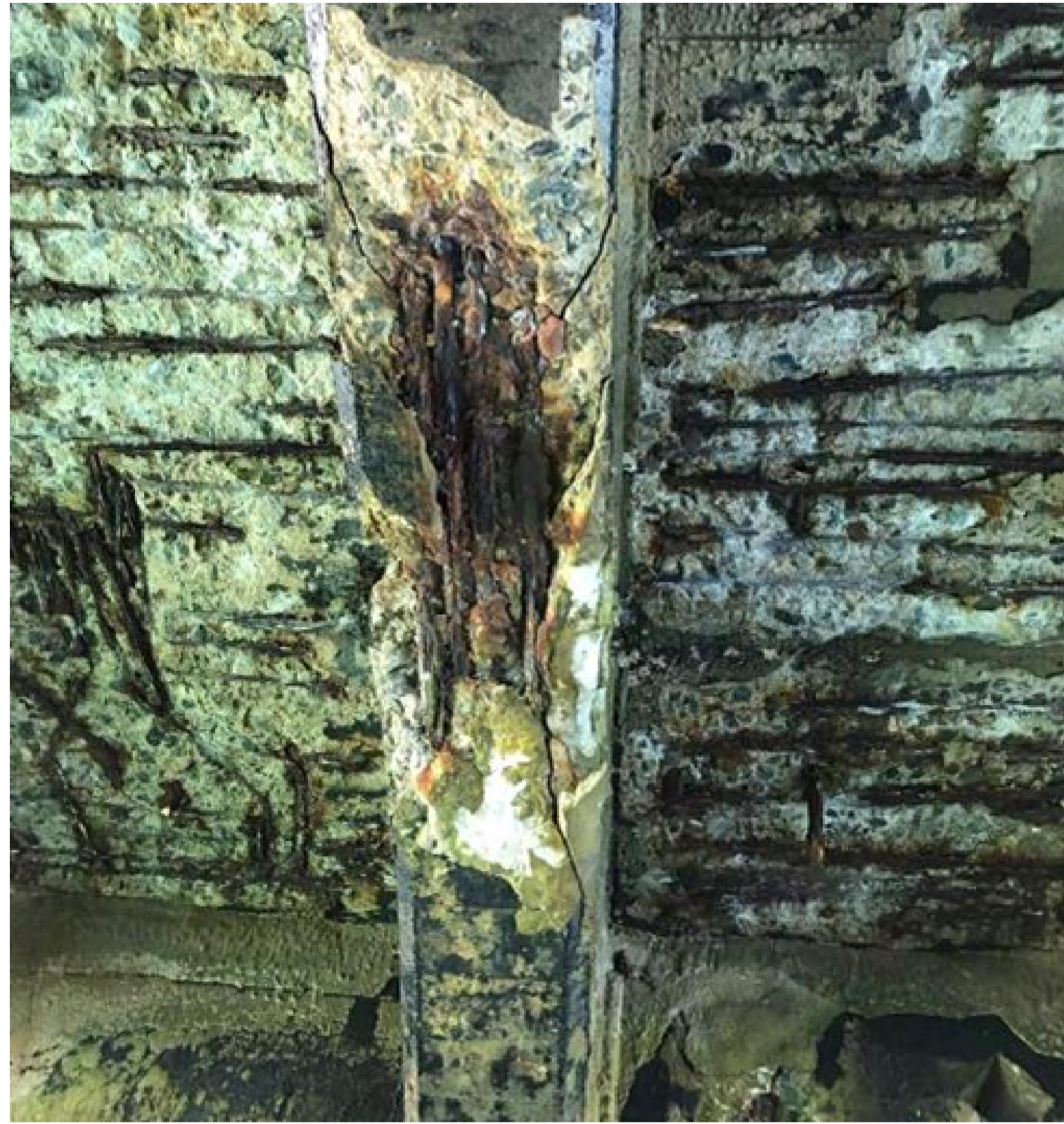
Photo 1 - Typical Cross Beam and Deck Soffit N.T.S.
