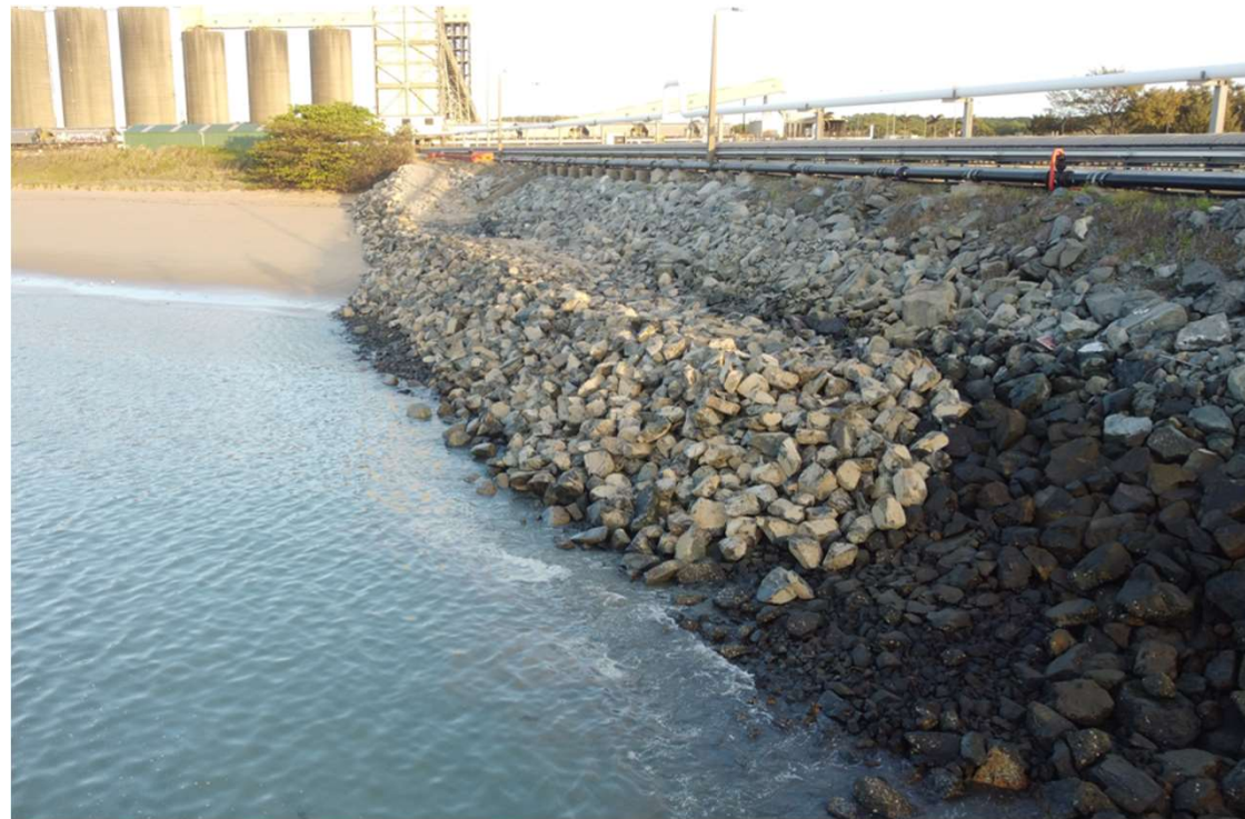
A temporary causeway has been built to facilitate the Northern Revetment repairs.
