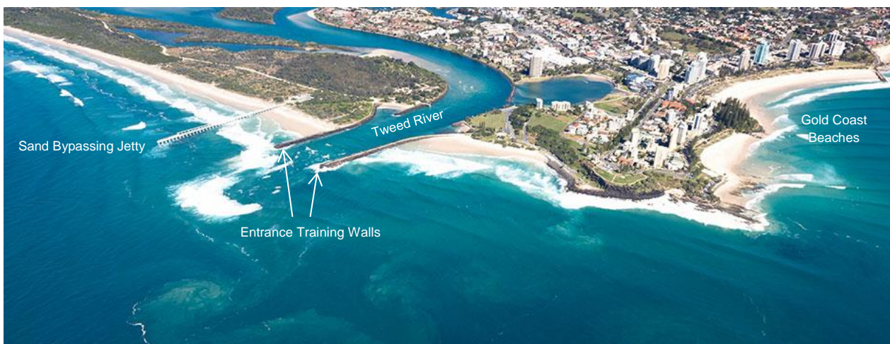
Figure A2: Entrance training walls and sand bypassing system at Tweed River, NSW (Image source: TRESBP, 2016)
