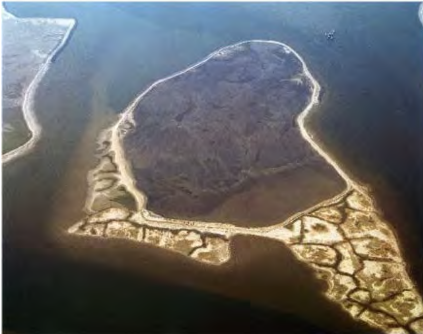
Figure 4-10 IJssel Delta offshore bund environmental area under construction
