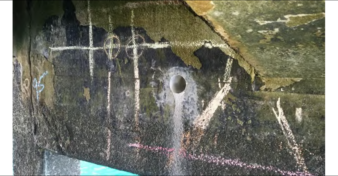
Breakout of upwards diagonal bar – 12 mm round (not deformed/ribbed)
