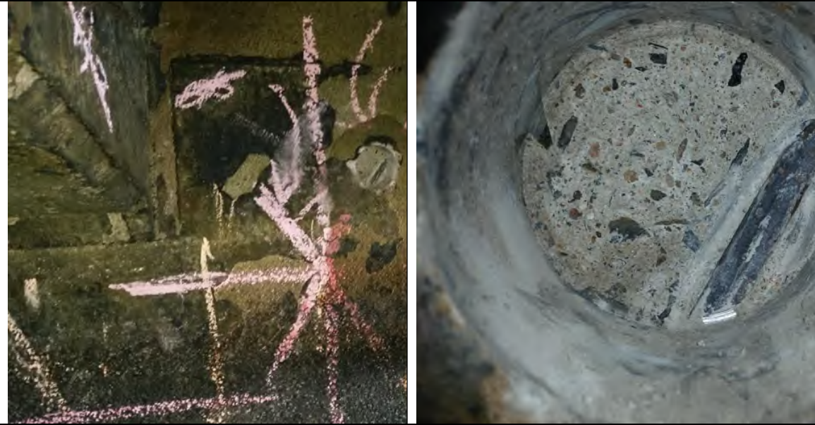
Breakout of upwards diagonal bar – 12 mm round (not deformed/ribbed)
