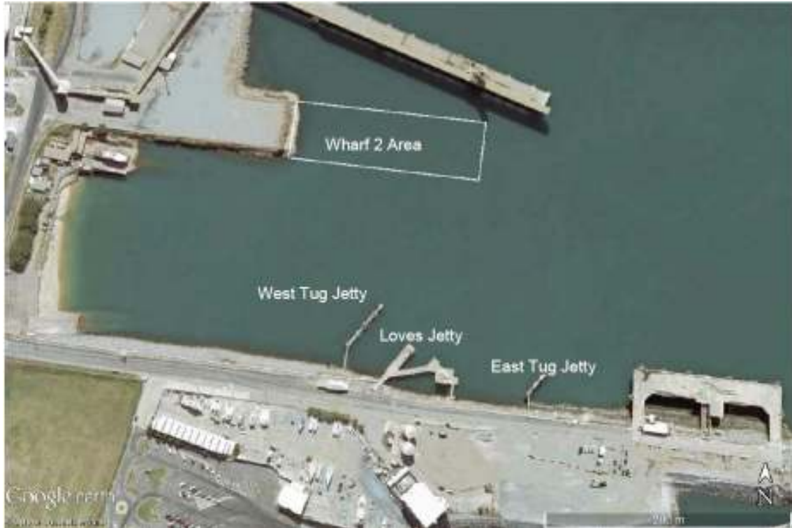
Figure 1 Structures Proposed for Demolition
