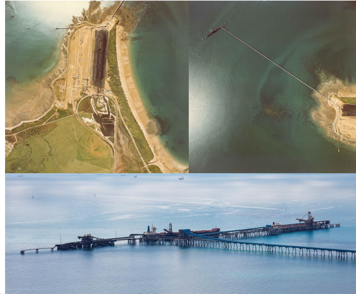
Hay Point Coal Terminal in 1974 (above right) and (right) in 2019.
