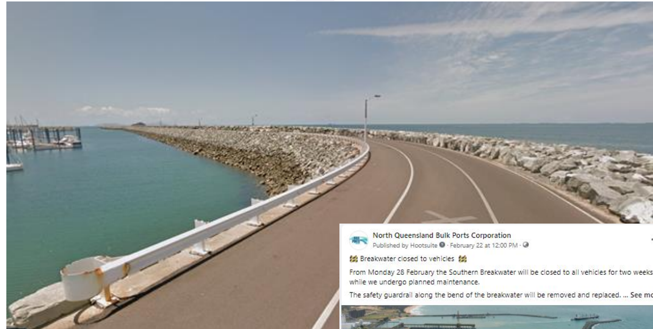
The safety guardrail along the bend of the Southern Breakwater is being replaced.
