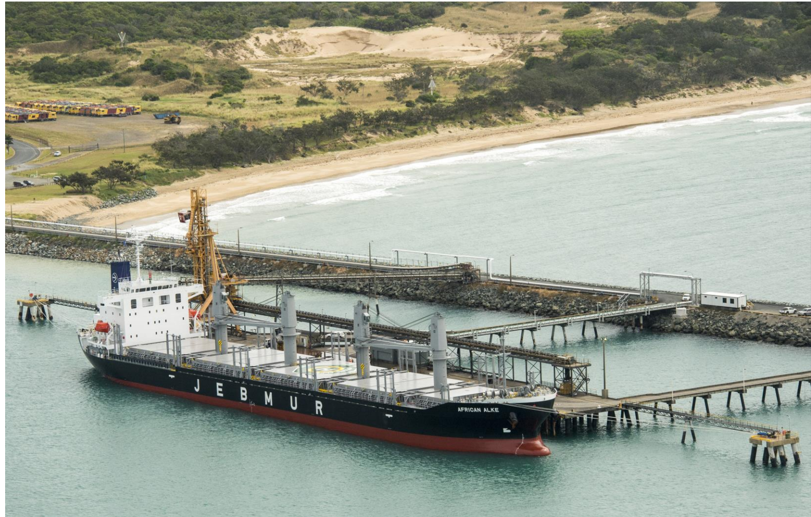
Tenders have been awarded for the Wharf 5 western access trestle replacement project.
