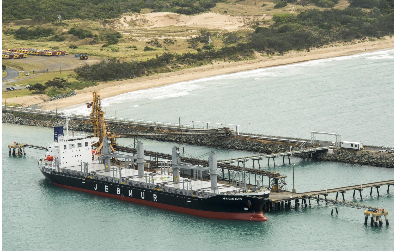
Tenders have been called for the Wharf 5 western access trestle replacement project.
