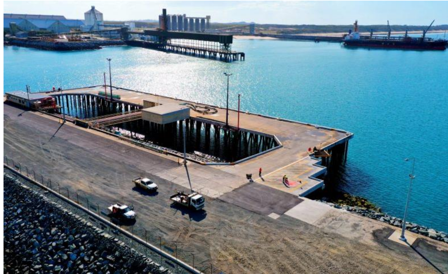
The Wharf 1 extension was completed in July 2021 VIDEO: https://www.youtube.com/watch?v=XKxfhyxUT7M
