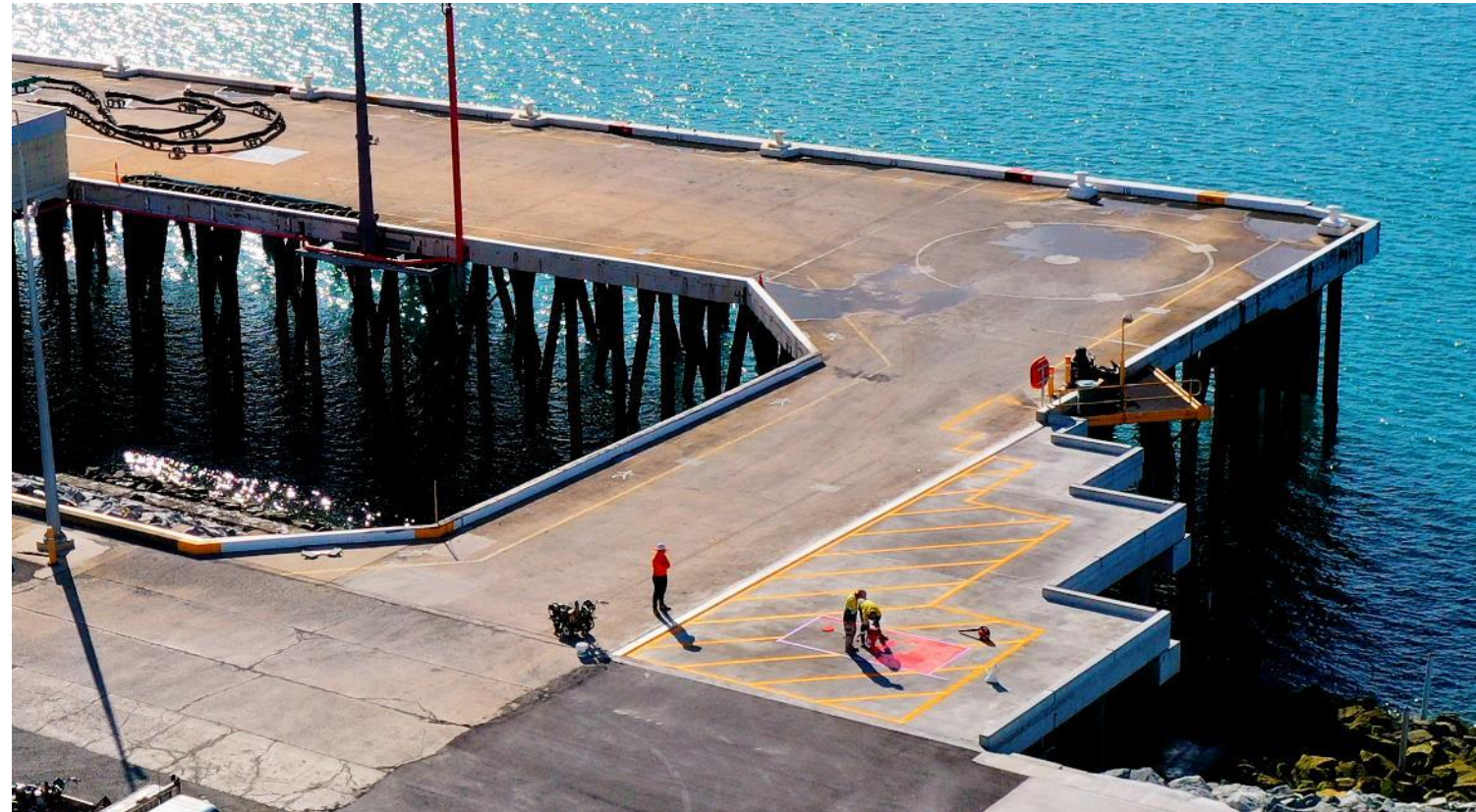
The Wharf 1 extension was completed in July 2021
