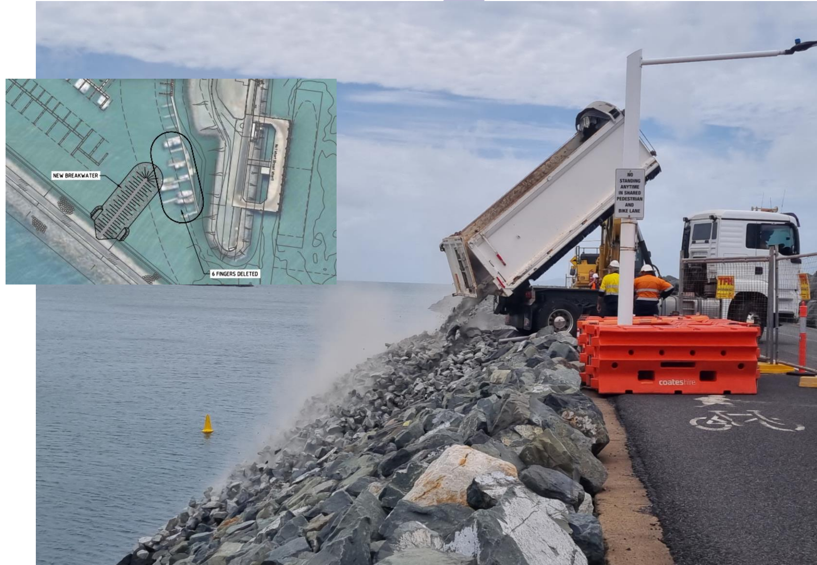
First truckload of rock unloaded for the construction of the Mackay Marina nib wall.
