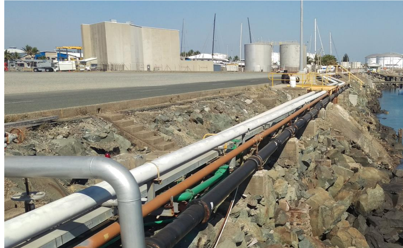
Existing alignment of fuel lines and services.
