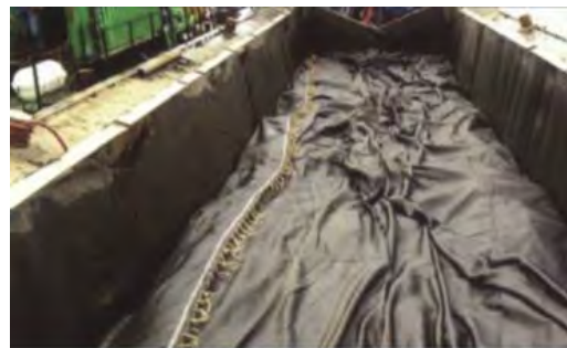
Figure 4-10: Geotube / geocontainer placement, source: TenCate (2016)
