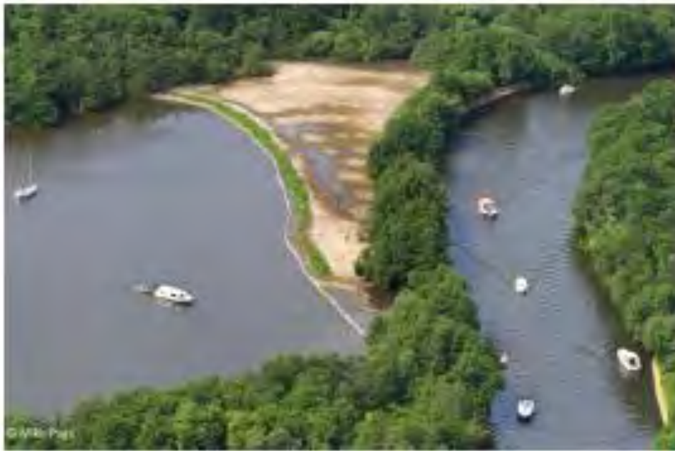
Figure 4-13: Mud flat habitat creation with bund at Salhouse Broad, UK, source PIANC Report No 176, 2018
