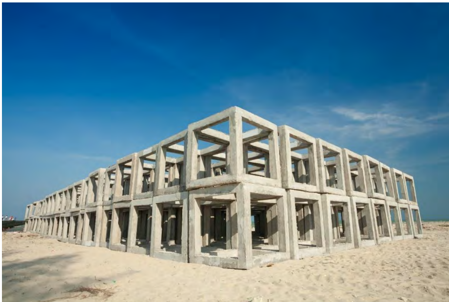
Figure 4-5: Example pre cast concrete unit for the creation of artificial reef
