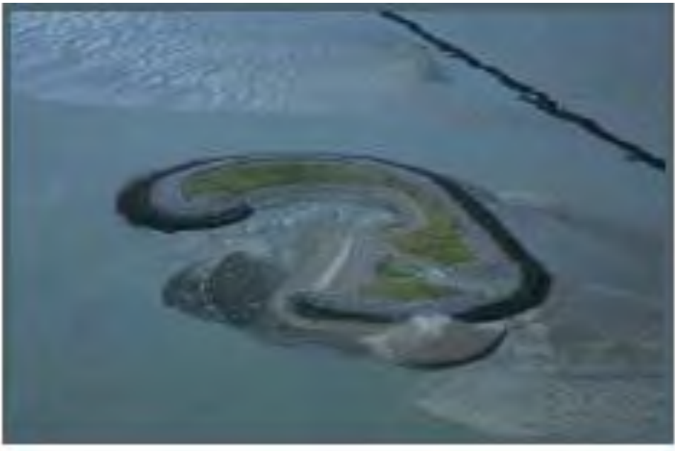
Figure 4-14: Bird island, Seine Estuary France constructed using offshore bund and dredged sediment, source PIANC Report No 176, 2018
