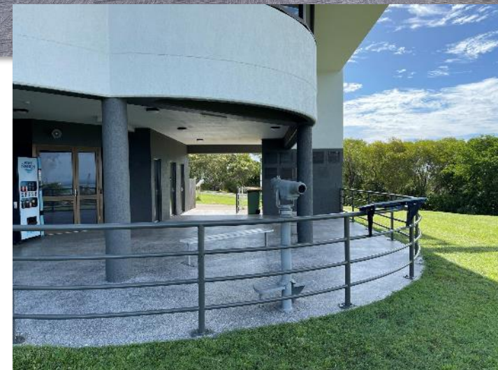
A new meeting room in the refurbished Hay Point Administration Building (top right) and public lookout area (right).
