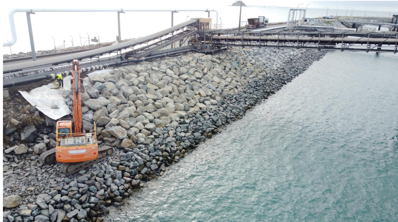
Works are progressing on the inner northern breakwater rehabilitation project.
