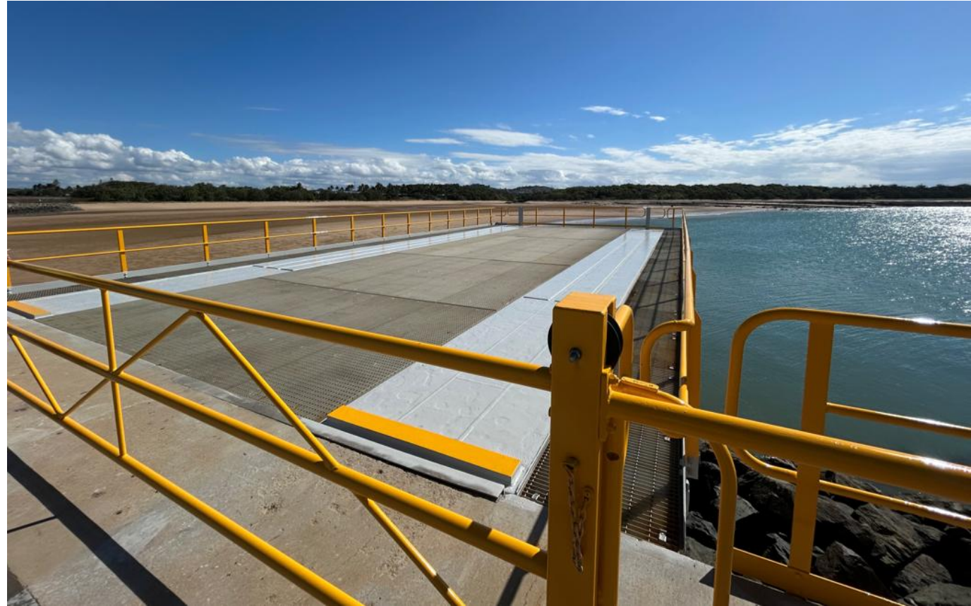
Maintenance works have been completed at the Half Tide MOF.
