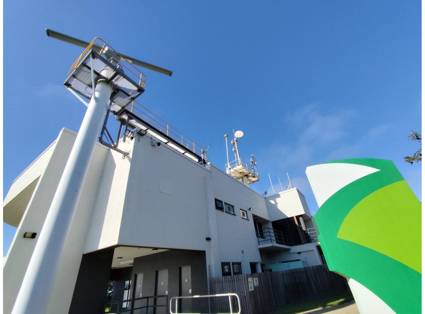
VTS Administration Building at Hay Point
