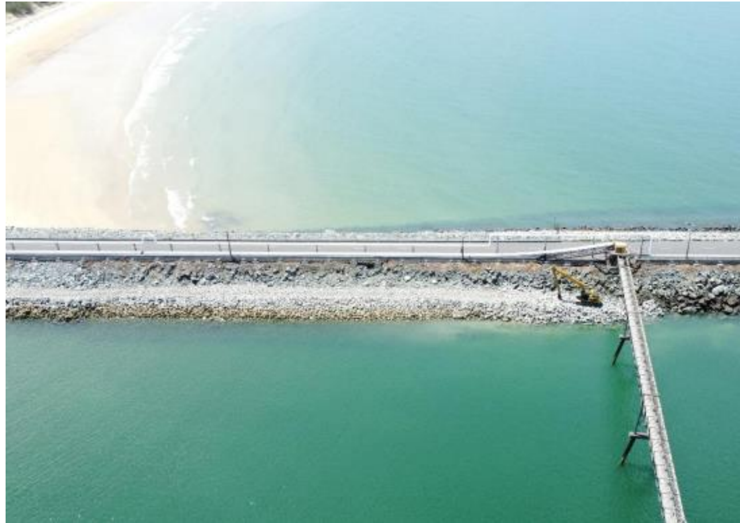
Works are progressing on the inner northern breakwater rehabilitation project.
