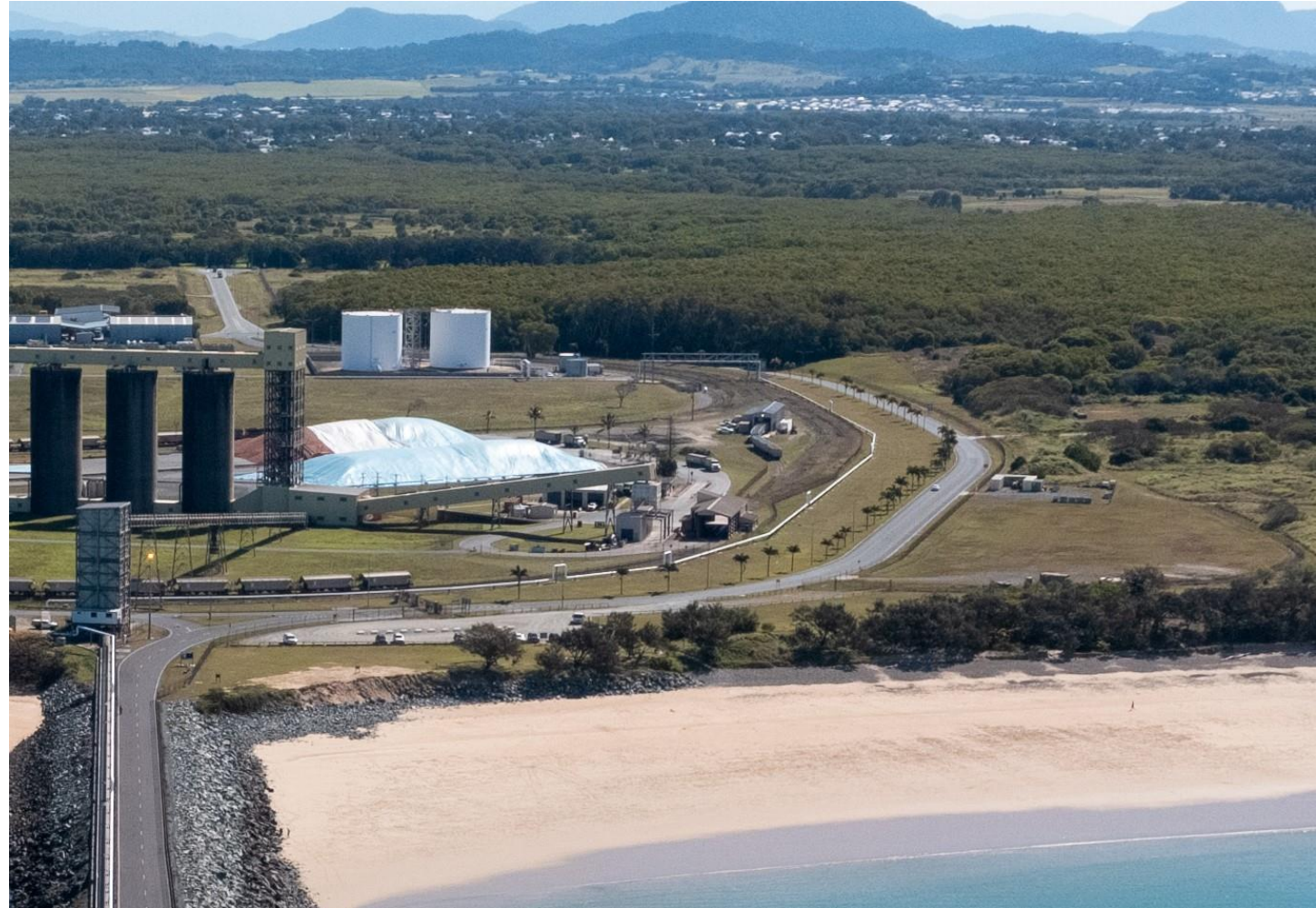
Aerial of North Wall beach
