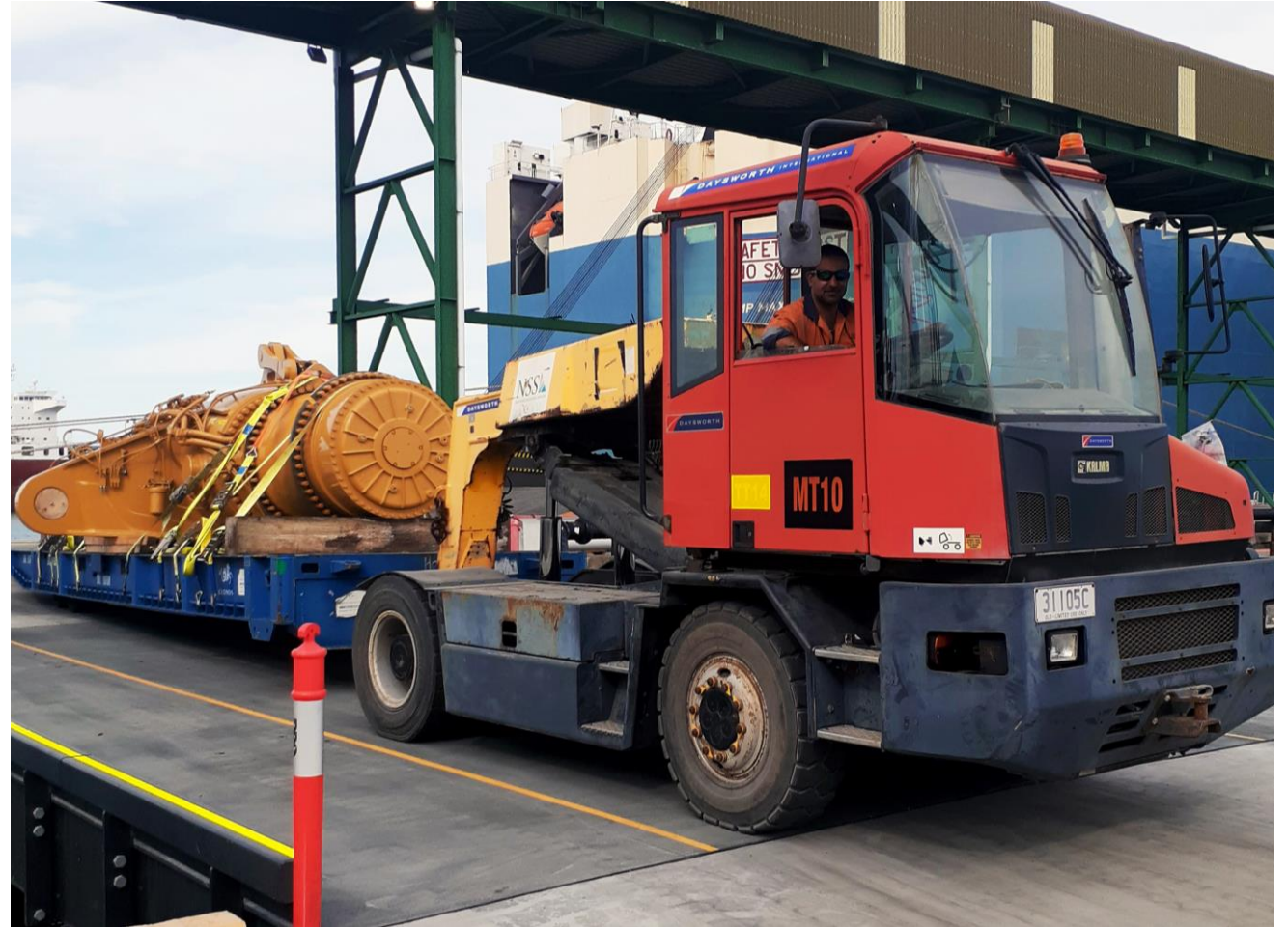
Above: The first equipment to come across the new Wharf 4 access deck.
