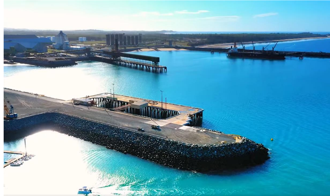
Port of Mackay’s Wharf 1 extension.
