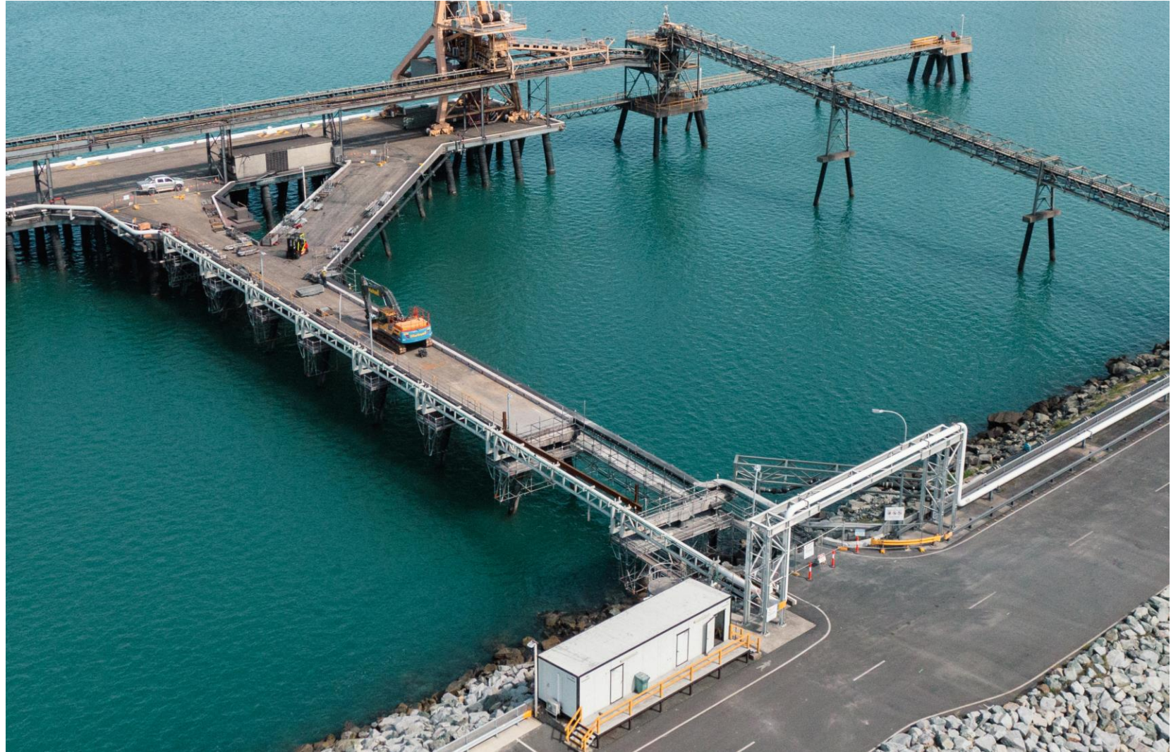
Works on the Wharf 5 western access deck have been progressing. Pictured: Aerial of the worksite showing removal of deck spans.
