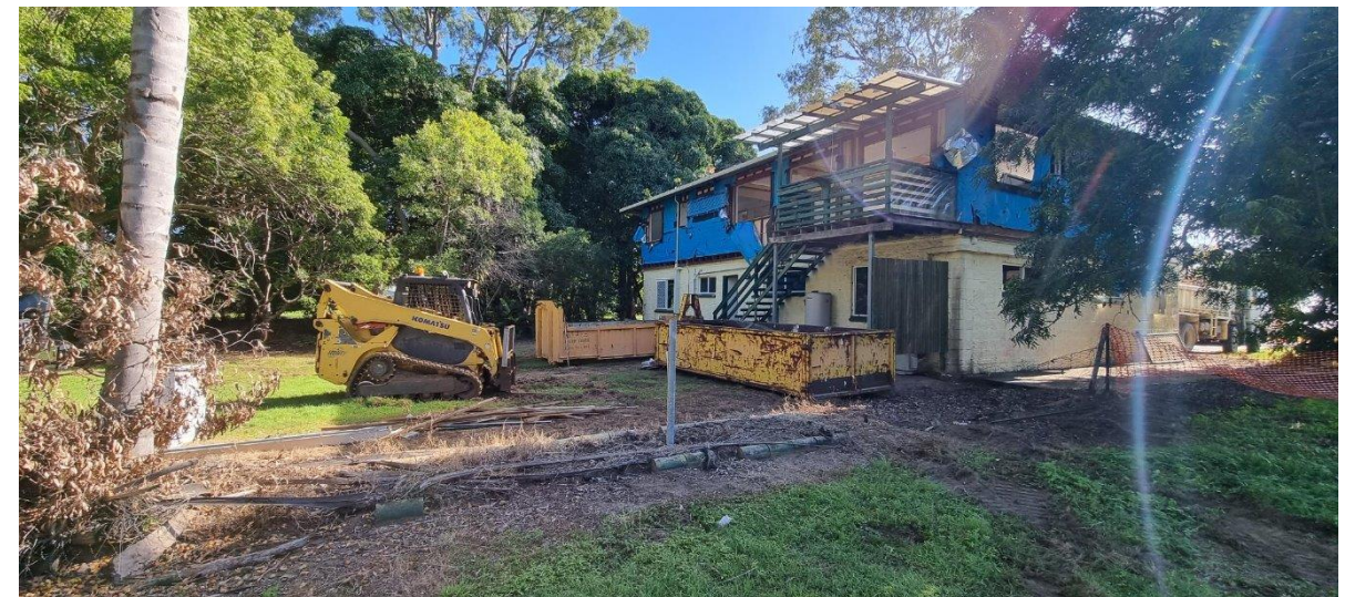
Demolition works at Louisa Creek - 2022
