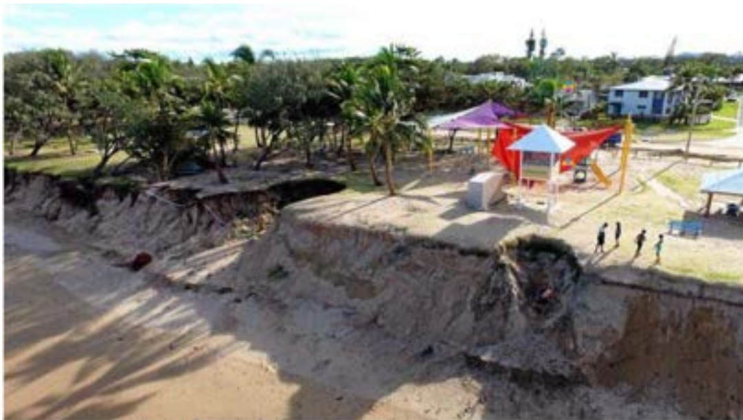
Figure 4-12 Beach erosion at Lamberts Beach (source: Michael Kennedy in Daily Mercury (19/09/17))
