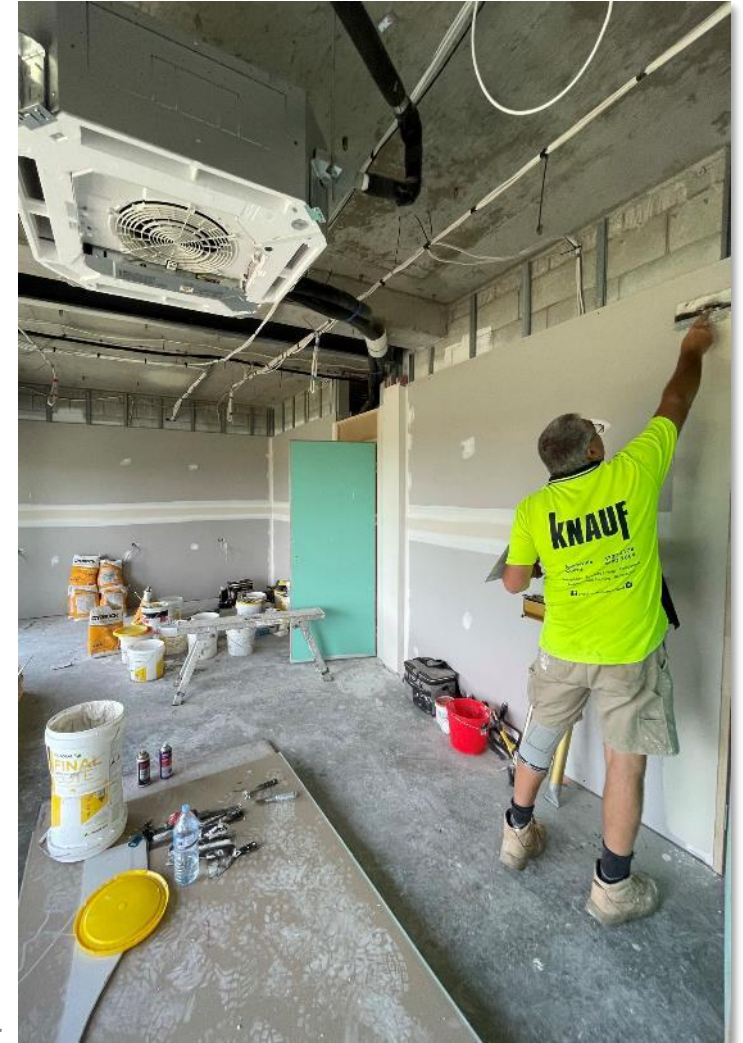
Internal fit outs continue at Hay Point Administration Building.
