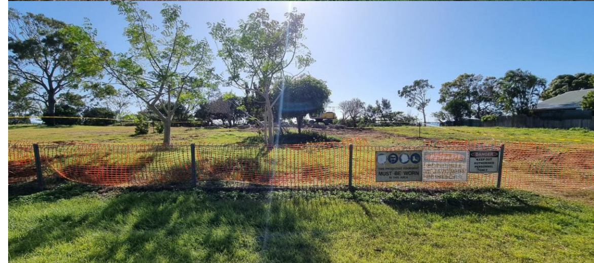
Demolition works at Louisa Creek.
