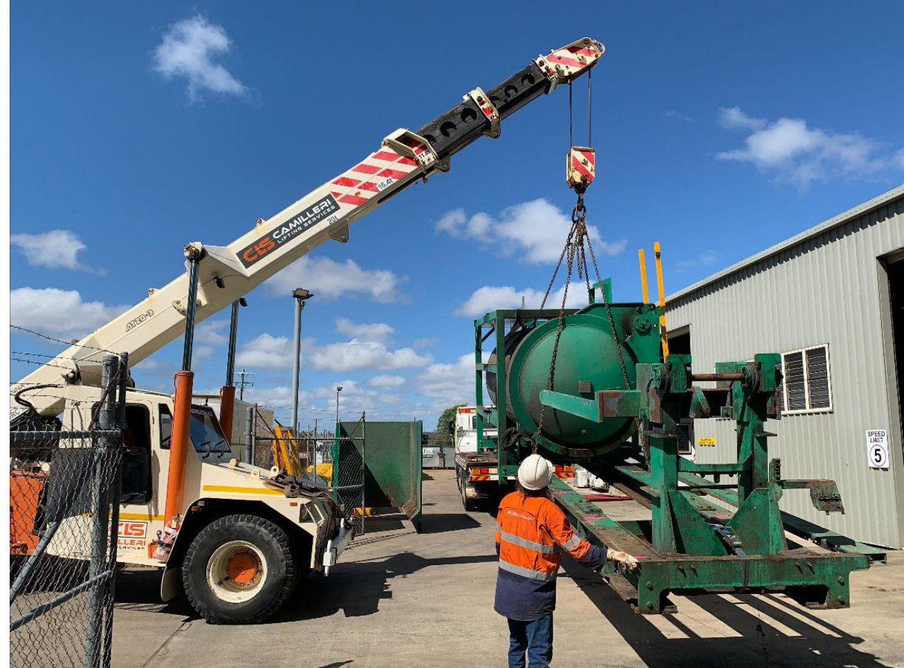
Above: Removal of an old autoclave from the Hay Point Quarantine Waste Facility.
