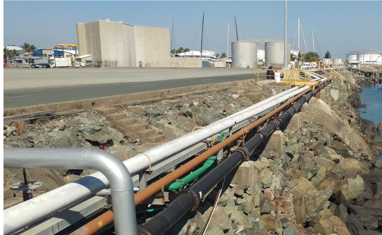
Existing alignment of fuel lines and services.
