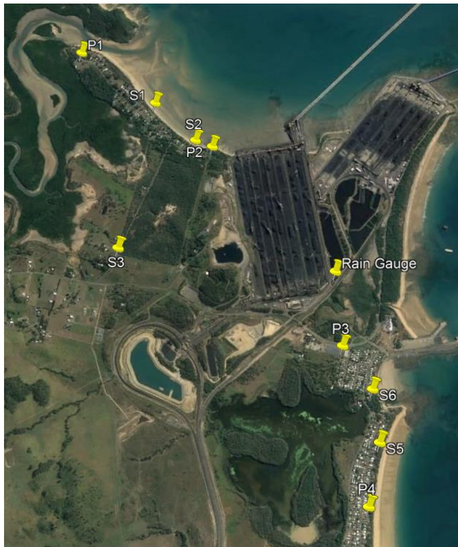
Figure 2: Detail of the Port of Hay Point Residential Stations Location and Rain Gauge
